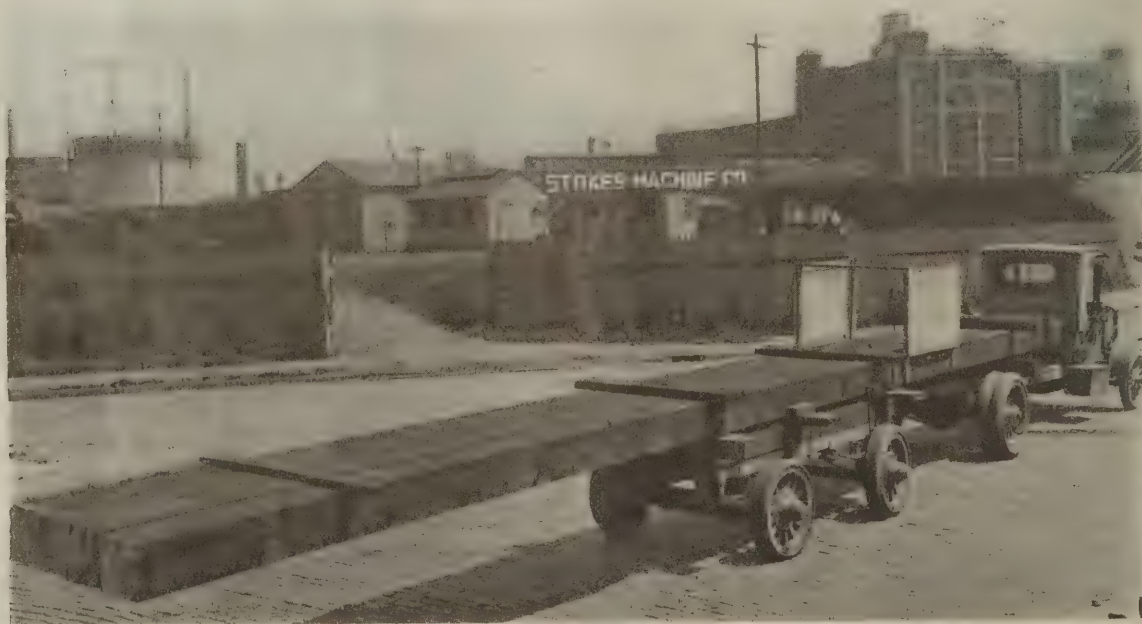
TRAILERS AS USED IN HAULING EXTREMELY LONG LENGTHS
